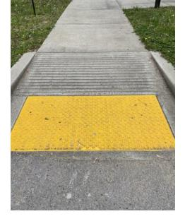
Curb cuts allow access from a parking area or road to the sidewalk. These tactile markers alert long cane users on the sidewalk that there is a hazard (a road!) is ahead. Photo: Freya McGregor.
